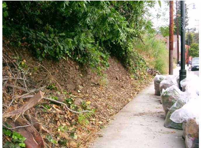
The Wall on Marmion Way
