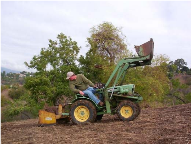
Luke Parker clearing away remains of the old fence line in Elyria.
